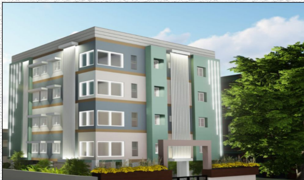
NAVARATHNA ORANGE RESIDENCY KK NAGAR, TRICHY.
