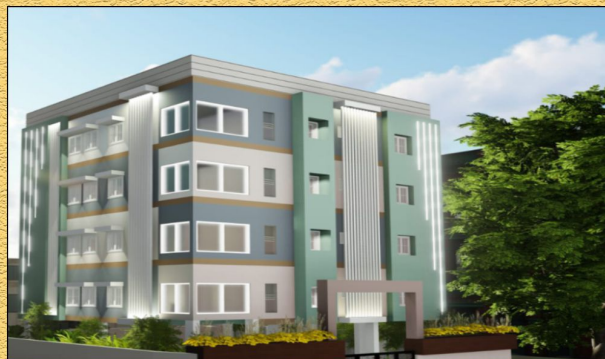
NAVARATHNA ORANGE RESIDENCY KK NAGAR, TRICHY.
